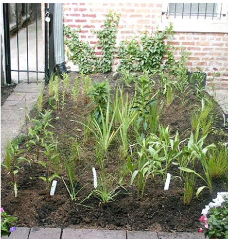
A rain garden catches rainfall and stormwater runoff and is designed to withstand the extremes of moisture and high concentrations of nutrients, particularly Nitrogen and Phosphorus that are found in stormwater runoff. Rain gardens catch stormwater runoff and serve to slow the stormwater as it travels downhill, giving the water more time to seep into the soil and less opportunity to gain momentum and erosive power.
