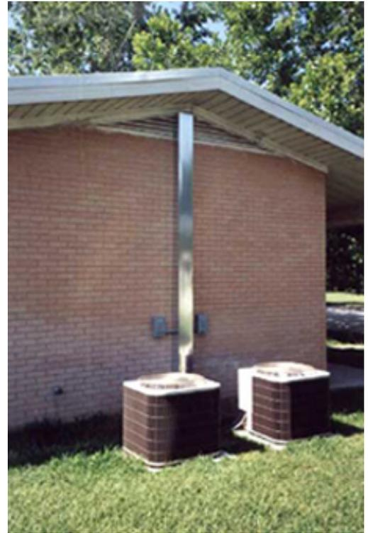
Central A/C units replaced inefficient window units and wall furnaces.
