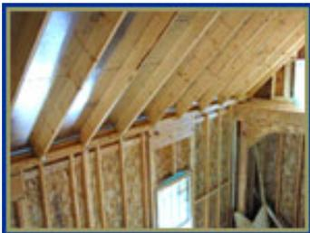
Value-engineered framing can reduce the amount of wood used in stick-frame construction as much as 25 percent.
