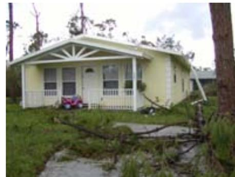
This affordable home in Florida withstood the damage of Hurricane Charley in 2004. It was built with fiber-cement-faced structural insulated wall panels and survived 145 mph winds. The insulated panels are also highly energy efficient.
