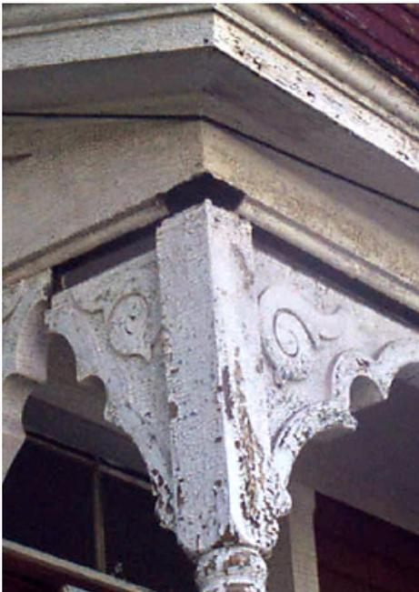
**FIGURE 1.2** Deteriorated residential paint on house trim.
