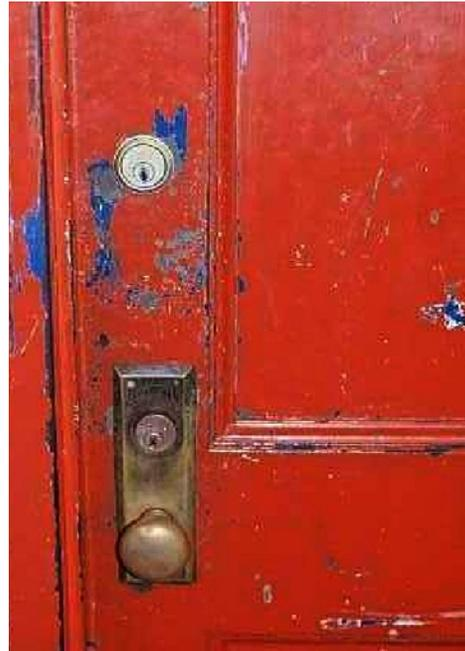
**FIGURE 1.3** Paint deterioration.
