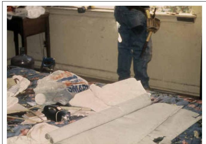
**FIGURE 4.3** This worksite was not properly prepared for lead-disturbing work by removing the occupant’s belongings.
