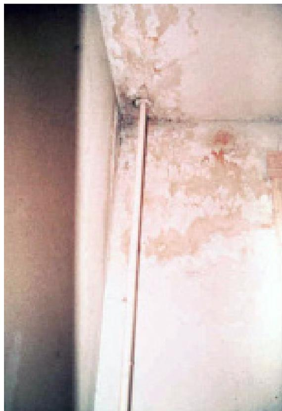
**FIGURE 13.2** Deteriorated paint on surfaces that are unsuitable for encapsulation
