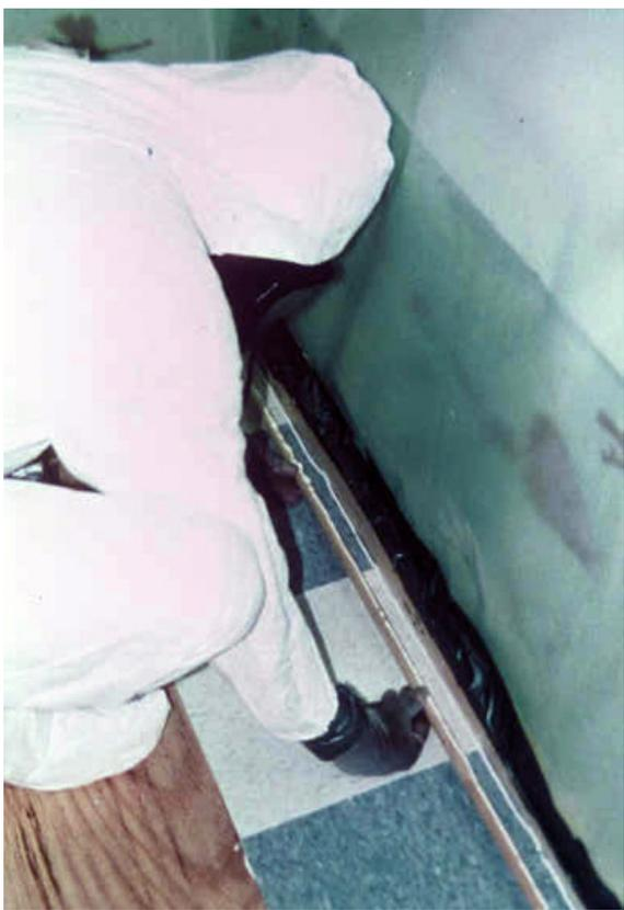
**FIGURE 13.1** Encapsulating a floor with vinyl tiles
